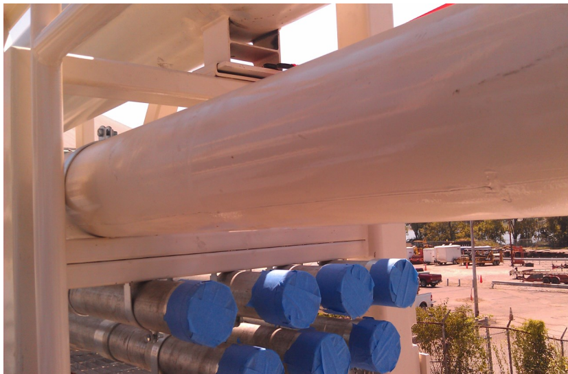
Modular System is Installed in 2 Days
