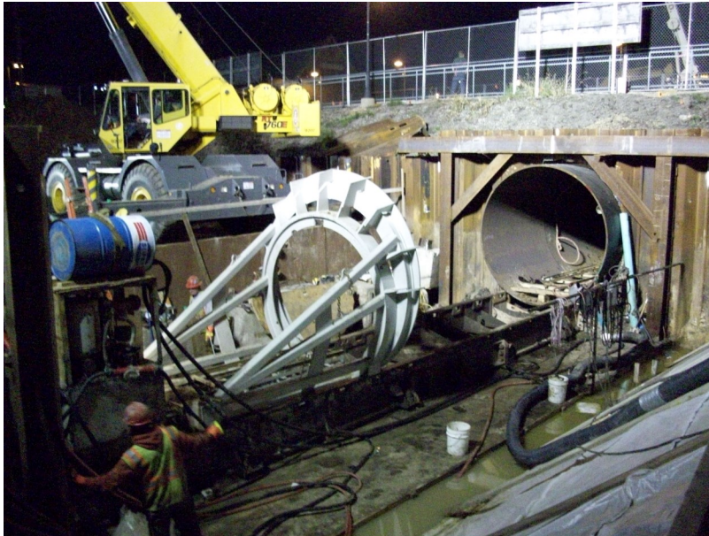
Innovative Technologies Allow Critical Tunnel Completion Under America's Busiest Railroad
