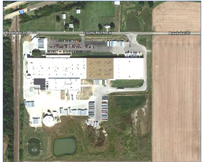
Plant expansion where Wishbone salad dressing is produced for the entire Midwest.
