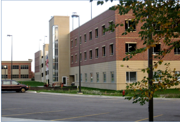
400 Car Parking Deck Structure
