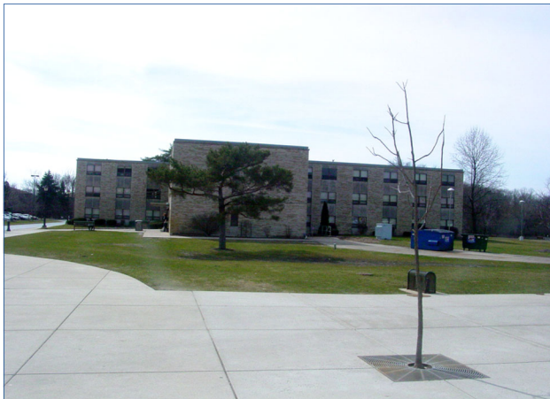
Smooth Project Delivery Results From Utility and Stormwater Planning
