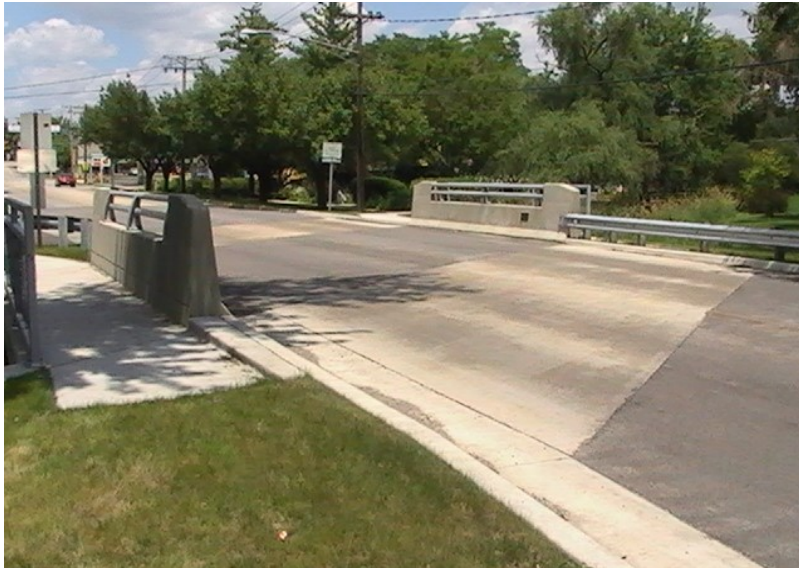
Fast track schedule constructed in town bridge reconstruction June-October, 2013.
