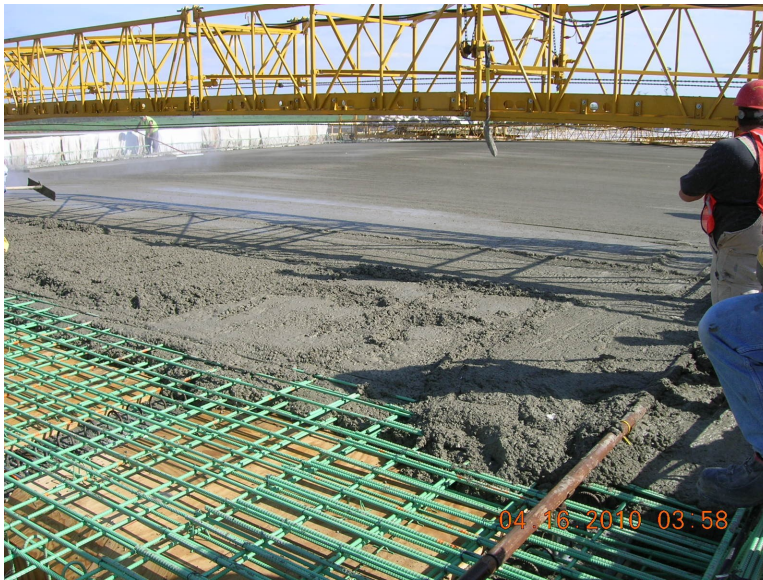
Tight quality control of deck pre-calculated dead load deflection to provide exact rail clearances required by Union Pacific Railroad.
