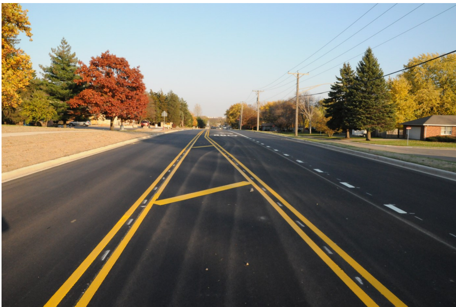
Upgraded Profile Grade Line Enhances Sight Distance and Traffic Safety
