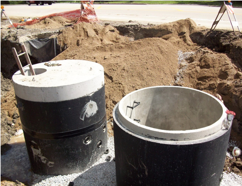
Sanitary Lift Station
