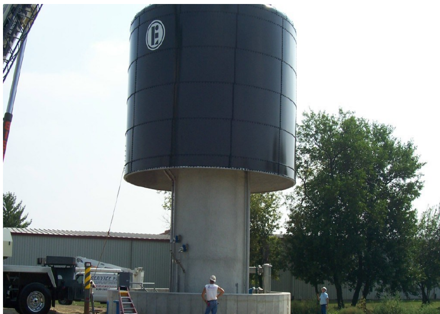
Radium Removal Plant
