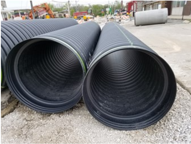
Upgraded Storm Sewer Outfall
