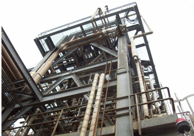
Allowed Dissolved Air Flotation Building Project To Meet Schedule and Budget
